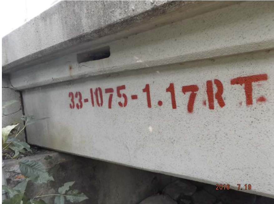
BRIDGE # - SPAN 1 - RIGHT
